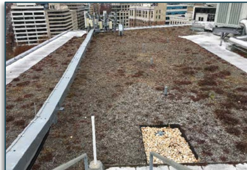
Figure 10 – Lafayette Building December 2018
