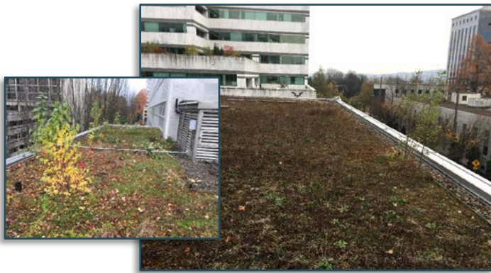
Figure 18 – 911 Federal Building November 2018
