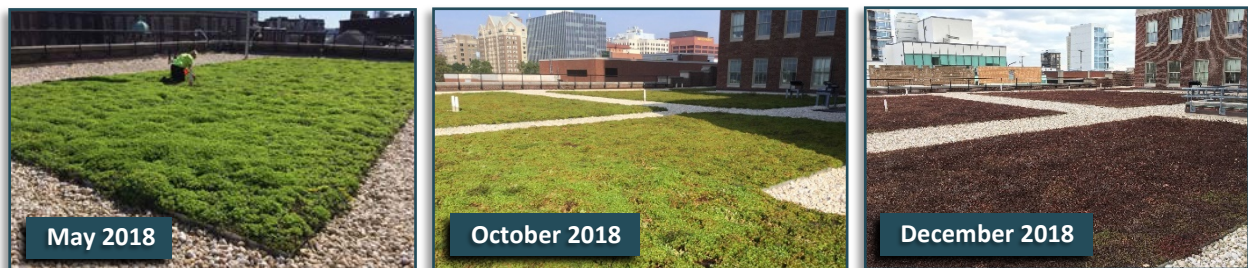
Figure 3 – U.S. Custom House Green Roof Seasonal Photographs
