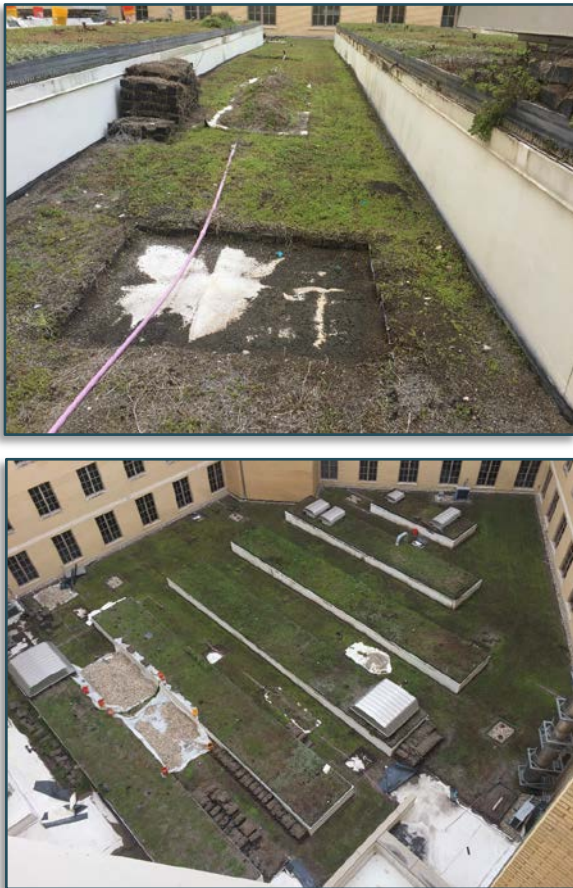
Figure 14 – Hipolito F. Garcia U.S. Courthouse December 2018
